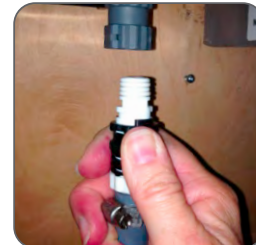
3. Detach flow jet hose from the cartridge.
